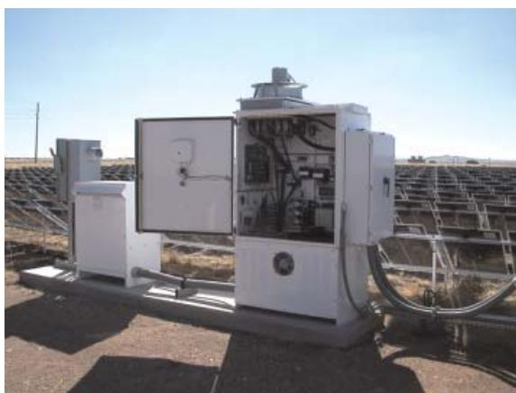
Figure 3. Xantrex PV150 system inverter
